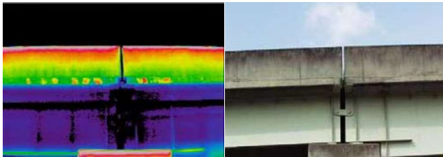
Diagnosis of structure (Bridge)
